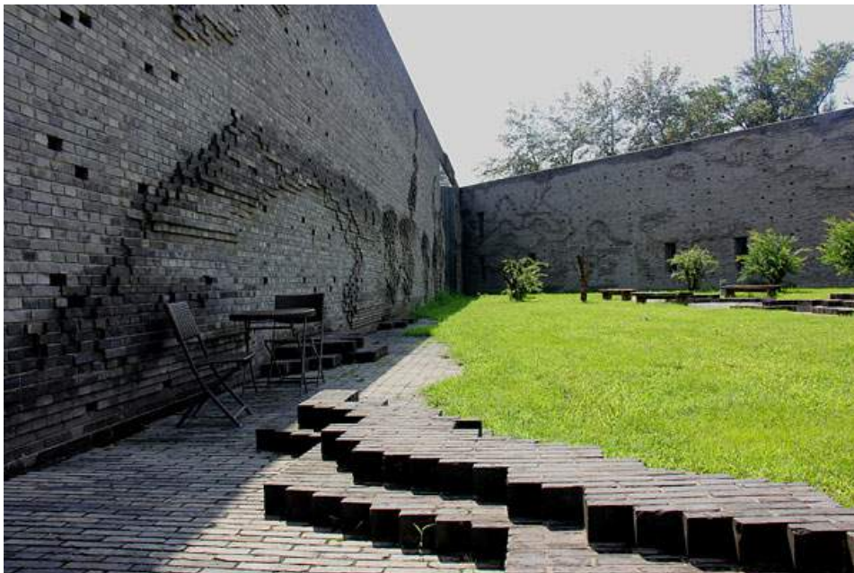
Fig. 16. Ai Weiwei, Three Shadows Photography Centre , The first institution for the exhibition and production of photography and video art, commissioned by Chinese photographer Rong Rong in 2006. His Studio was a prototype for the architectural design.
